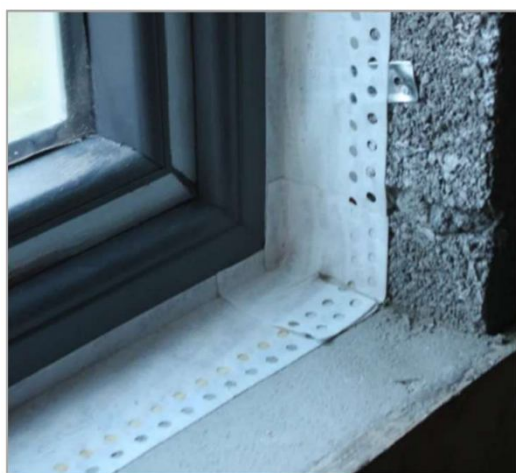
Figure 3: Air tight taping around window ope
